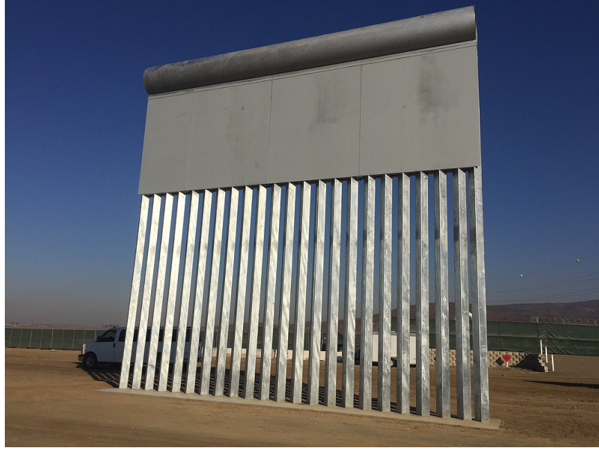
Figure 3.1: One of the prototypes built for the UMBW.
